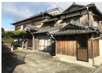
Vacant homes exist but are not being utilized.
